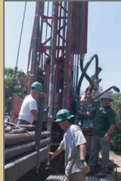
Hoisting core barrel up to line up over wireline casing
