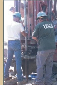
Core barrel being tripped down hole
