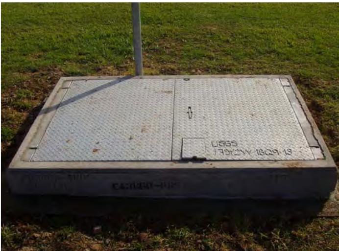
Figure 3E. Typical final installation of 3 by 5 foot, trafficked vault. USGS and well ID are welded on top of vault.
