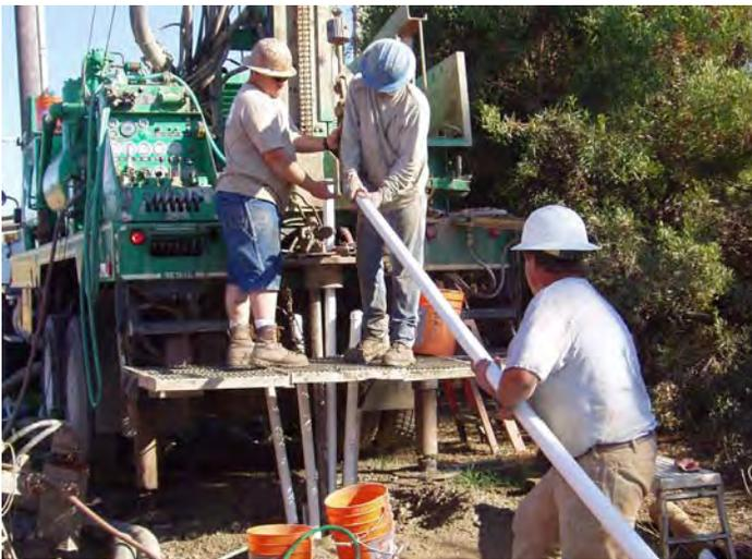
Figure 3B. Installation of 2-inch PVC pipe which will allow access to specific depths to measure water levels and sample water quality. Note 3 other piezometers are installed already.
